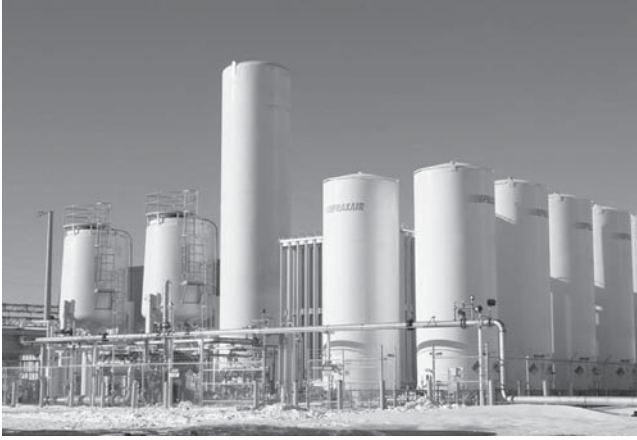
Figure 15.11. VPSA Plant; 180t/day; Amarillo, TX (photo courtesy of Praxair) Praxair is a registered trademark of Praxair, Inc.
