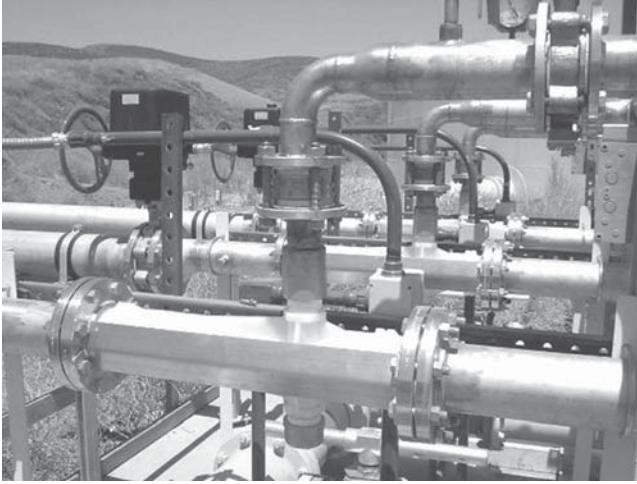
Figure 15.21. Ozone injector.
