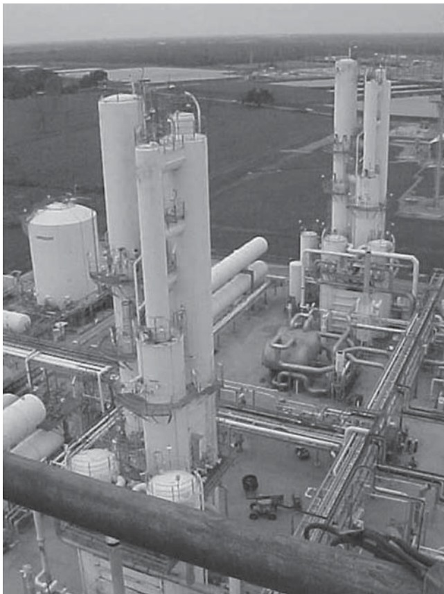
Figure 15.14. Cryogenic air separation facility; 6500t/day, East Chicago, IN (photo courtesy of Praxair) PRAXAIR is a registered trademark of Praxair, Inc.
