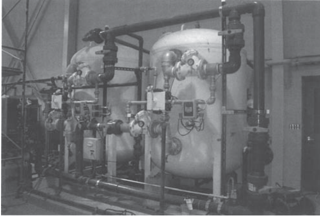
Figure 10.5. Typical duplex softening unit (courtesy of Black & Veatch).
