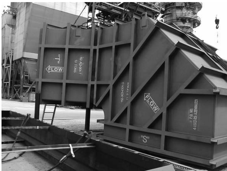
FIGURE 17.19 Duct containing static mixers and ammonia injection lances for SCR. (With permission from Haldor-Topsoe, Inc.)
