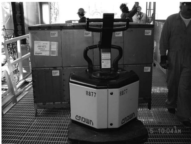
FIGURE 17.17 Pallet mover used to place SCR modules. (With permission from Haldor-Topsoe, Inc.)
