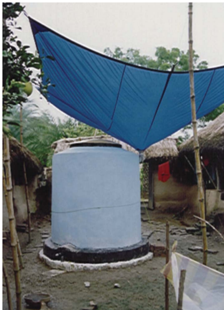
Chapter 14, Figure 7 Plastic sheet catchment for rainwater harvesting.
