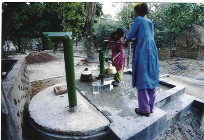
Chapter 14, Figure 4 Water collection from a protected (covered) dug well.
