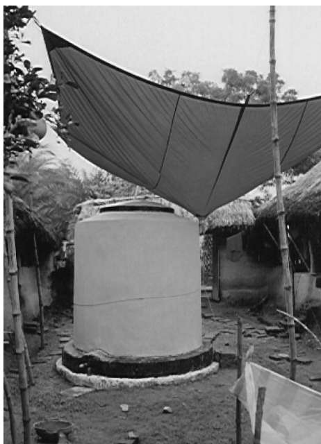
Figure 7 Plastic sheet catchment for rainwater harvesting. (See insert for color representation of figure.)
