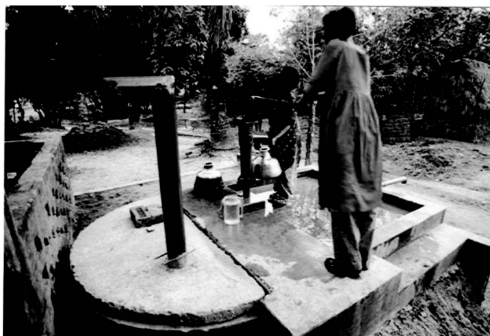
Figure 4 Water collection from a protected (covered) dug well. (See insert for color representation of figure.)
